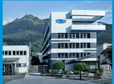
TYROLIT headquarters in Schwaz (Austria)
